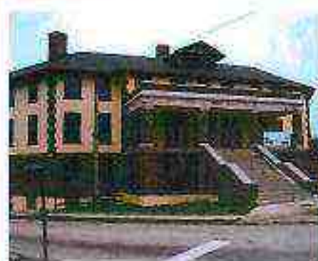
Exterior of the Inn with a new roof and fresh coat of paint.
